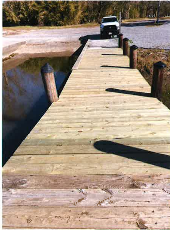
Replaced Substandard Pier Decking
